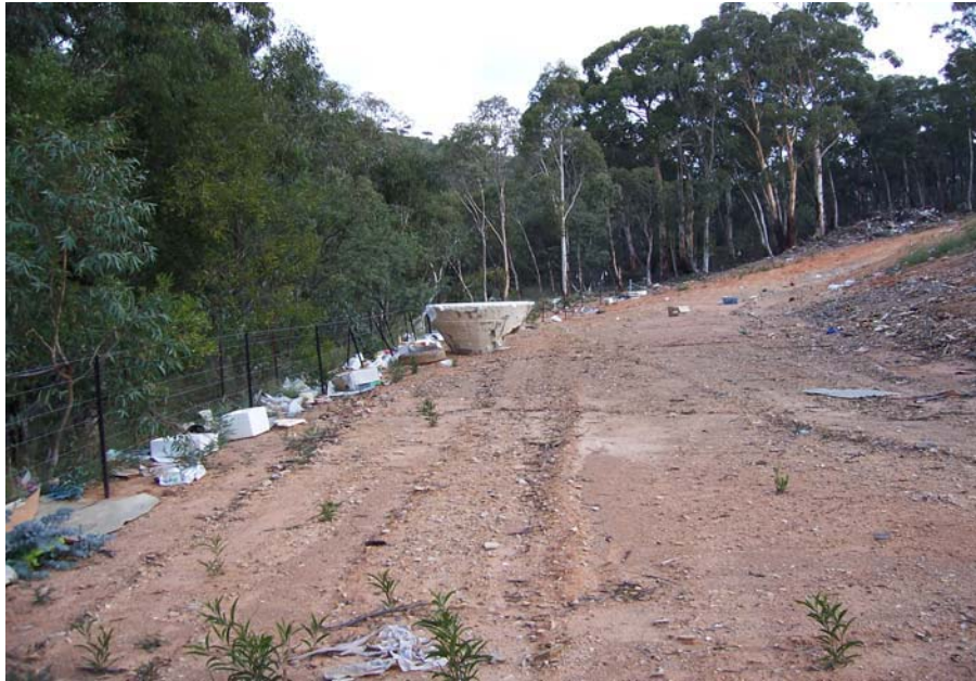
Photo 11: Windblown litter against landfill fence and into adjoining properties
