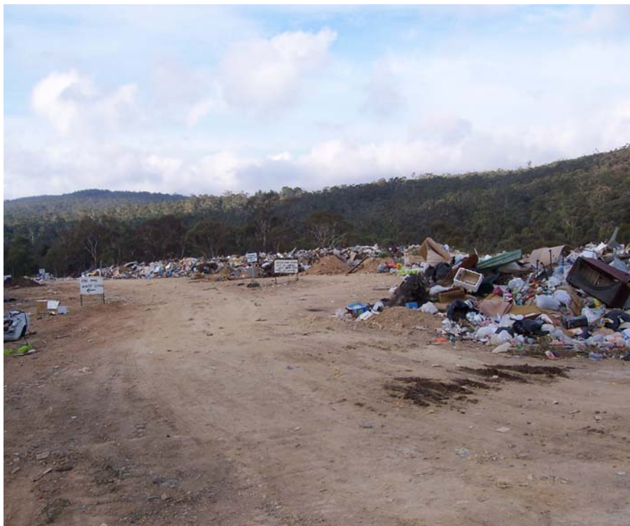
Photo 12: Waste kept uncovered for long periods (greater than 2 weeks) due to unavailability of cover material resulting in windblown litter, feral animals, odour and increased leachate.
