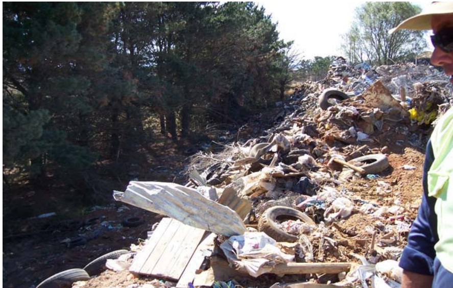
Photo 3 Uncovered batter slope
